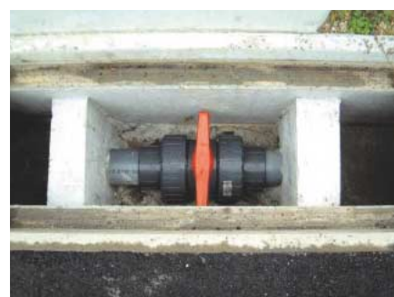
Example of emergency containment structure
