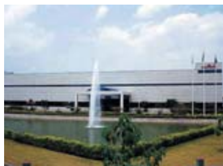
Murata Electronics (Thailand), Ltd.
