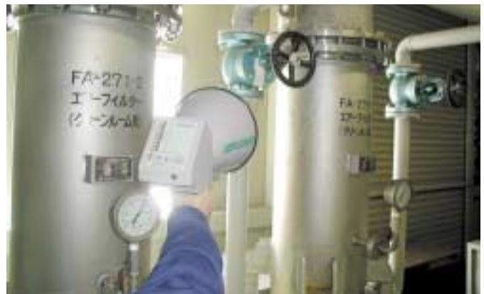
Inspection for leakage of compressed air
