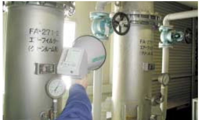
Inspection for leakage of compressed air
