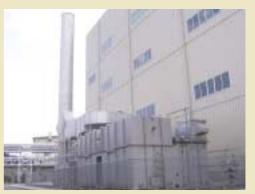
Regenerative Thermal Oxidizer (Fukui Murata Manufacturing Co., Ltd.)
