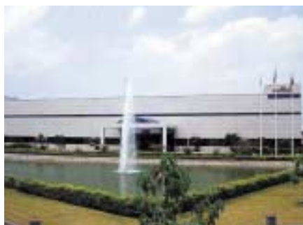
Murata Electronics (Thailand), Ltd.
