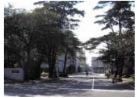
Murata Manufacturing Co., Ltd. Yokaichi Plant
