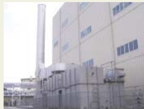
Regenerative thermal oxidizer (Fukui Murata Manufacturing Co., Ltd.)
