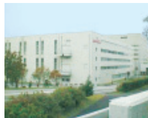
Kanazawa Murata Manufacturing Co., Ltd.
