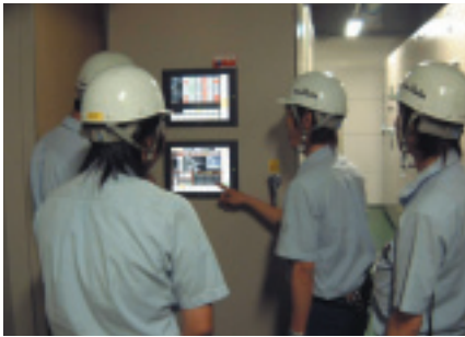
Monitoring of cogeneration system operations
