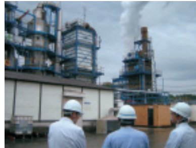
Inspection of industrial waste disposal company
