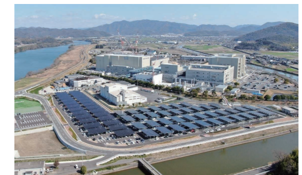
Parking lot-style mega solar system at Okayama Murata Manufacturing Co., Ltd.
