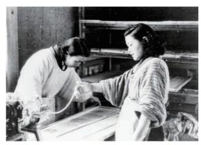
Production of titanium-dioxide ceramic capacitors
